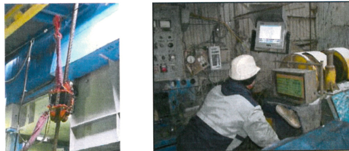
Fig.3. Inspection of 26 mm drilling rig.
