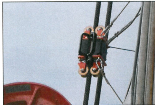
Fig. 2. INTROS-AUTO inspects 35 mm rope at drilling rig in Czech Republic.
