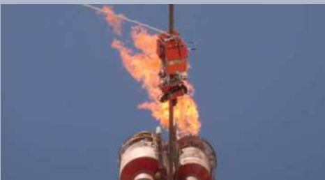
INSPECTION OF FLARE STACK GUY ROPES
