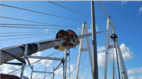
MRT OF BRIDGE CABLES
